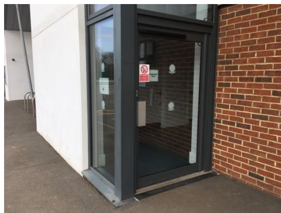
The sports pavilion doors are at ground level so there is no trip hazard and easy wheelchair access
